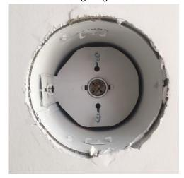
These areas are often neglected because it is unclear which subcontractor is responsible for doing the work. To avoid this problem, assign the entire task of post-drywall air sealing to a specific subcontractor in their scope of work. Instead of making each trade responsible to caulk around drywall penetrations during trim out, have the painter or the drywall installer do the air sealing all at once. This method gives the site supervisor a single trade to hold accountable for the work.
