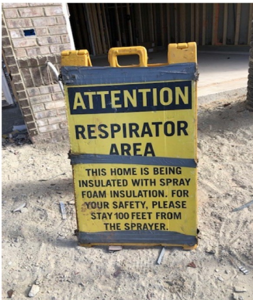
Sign warning of health hazards
