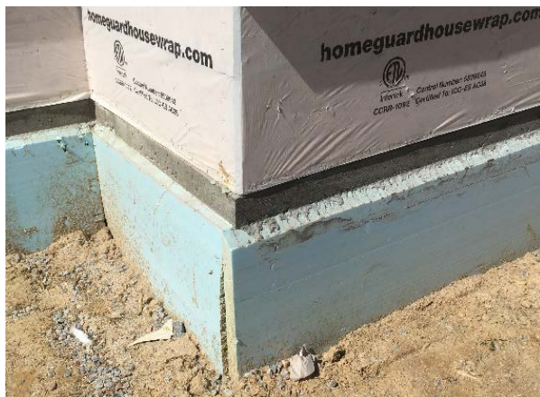
Monolithic slab insulation
