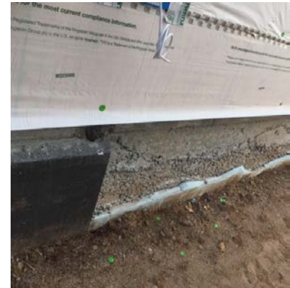
A large portion of removed slab insulation.
