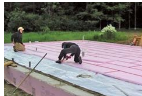
Under slab insulation example
