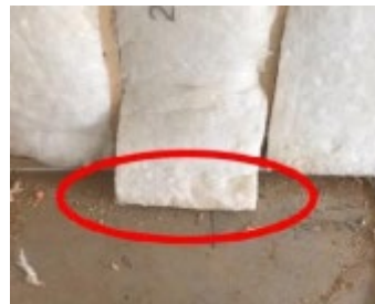
Insulation cut long and rolled at the bottom.
