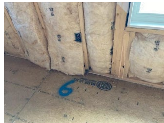
Insulation with compression greater than \frac{3}{4} ".
