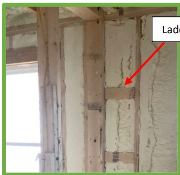
Ladder framing that allows the entire wall cavity to be insulated
