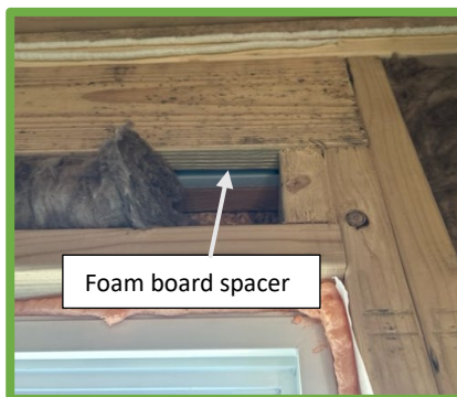
An advanced framed 2x4 wall with foam board.
