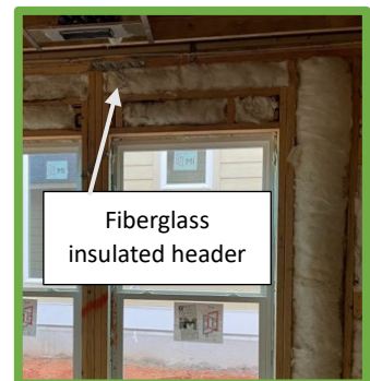
An advanced framed 2x6 wall with fiberglass insulation.
