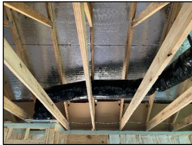
Radiant barrier, baffling installed correctly.
