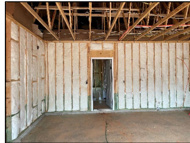
Insulation dam at the garage installed properly.
