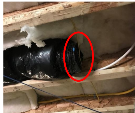
Examples of unconnected ducts in the attic and crawl space
