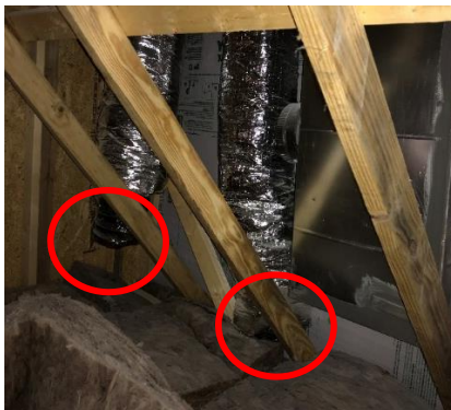
Examples of unconnected ducts in the attic and crawl space
