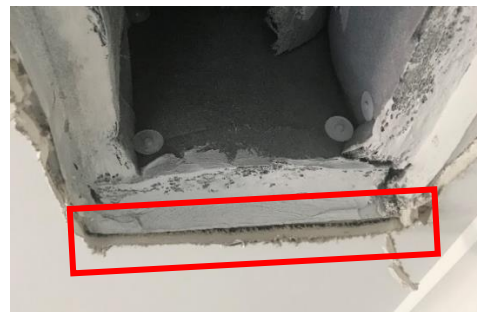
Examples of an unsealed supply and return
