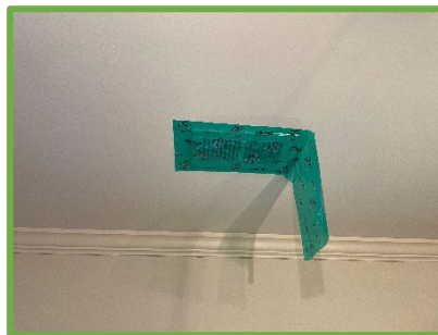
Tape covers supply and is sealed to the drywall.
