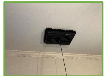
Vent cap covers the supply and seals to the drywall.
