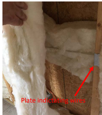
An example of an overfilled cavity with a plate highlighting the wire location
